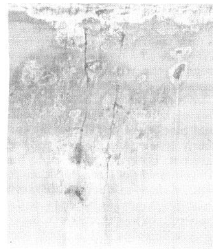
The wet spot on this lead keel indicates a pocket of porous material
